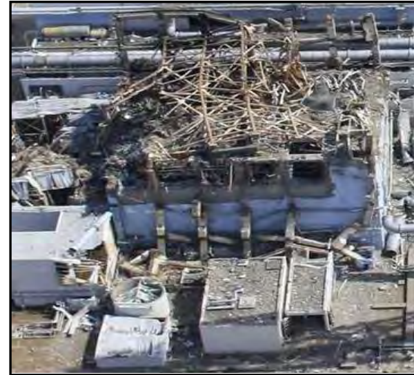
The severely damaged RB of U3 due to the hydrogen explosion (Source: TEPCO)
